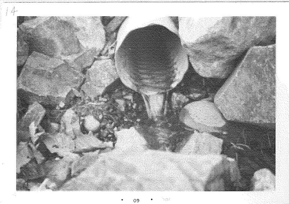
Photograph 14, shows the outlet of 8-inch perforated drain pipe laid at base of rock wall counter balance to remove subsurface water.
