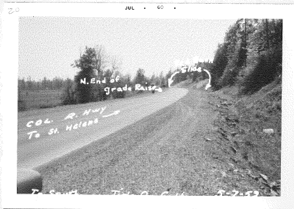
Photograph 20 shows the completed grade raise, counter balance and slide area.
