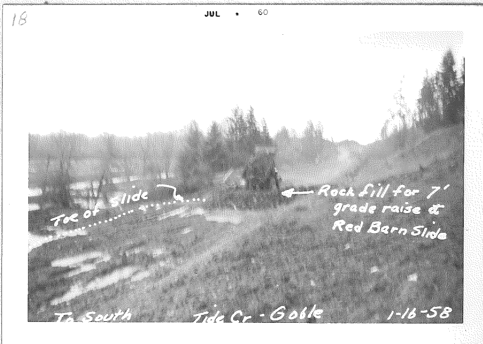
Photographs 18 and 19 show the corrective action taken to counter balance the slide.
