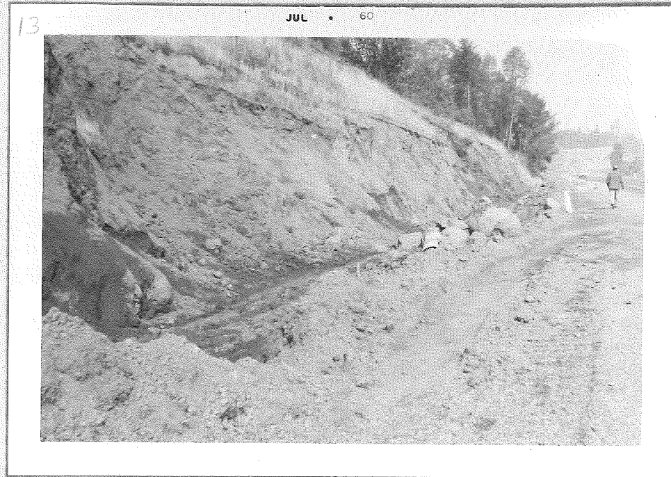
Photograph 14, shows the outlet of 8-inch perforated drain pipe laid at base of rock wall counter balance to remove subsurface water.
